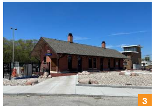
1. Ravenswood Station Rehabilitation 2. Grayland A32 Bridge Replacement 3. Blue Island Station Reconstruction
